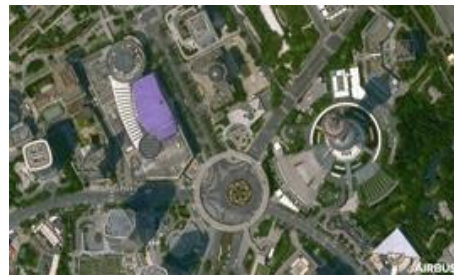
Shanghai Tower, Shanghai, China
